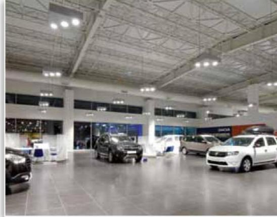
Lighting of other Renault automobiles available in the sales area involved custom-made 2x40W LED pendants which are placed especially to avoid flashing of light on top of the automobile while allowing for glowing from the sides. Built on a very large area, the distributor required its corridor areas to have lower illuminance levels when compared to the other areas with 2x20W LED pendants for its customers to visit the showroom in comfort.
